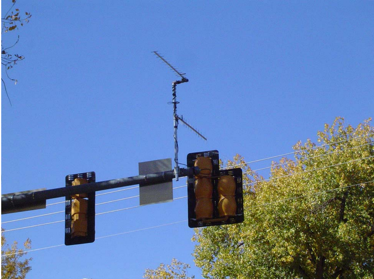
Figure 1 Yagi-Uda Antennas on Traffic Lights (Courtesy of Mr. J. Wolf)
